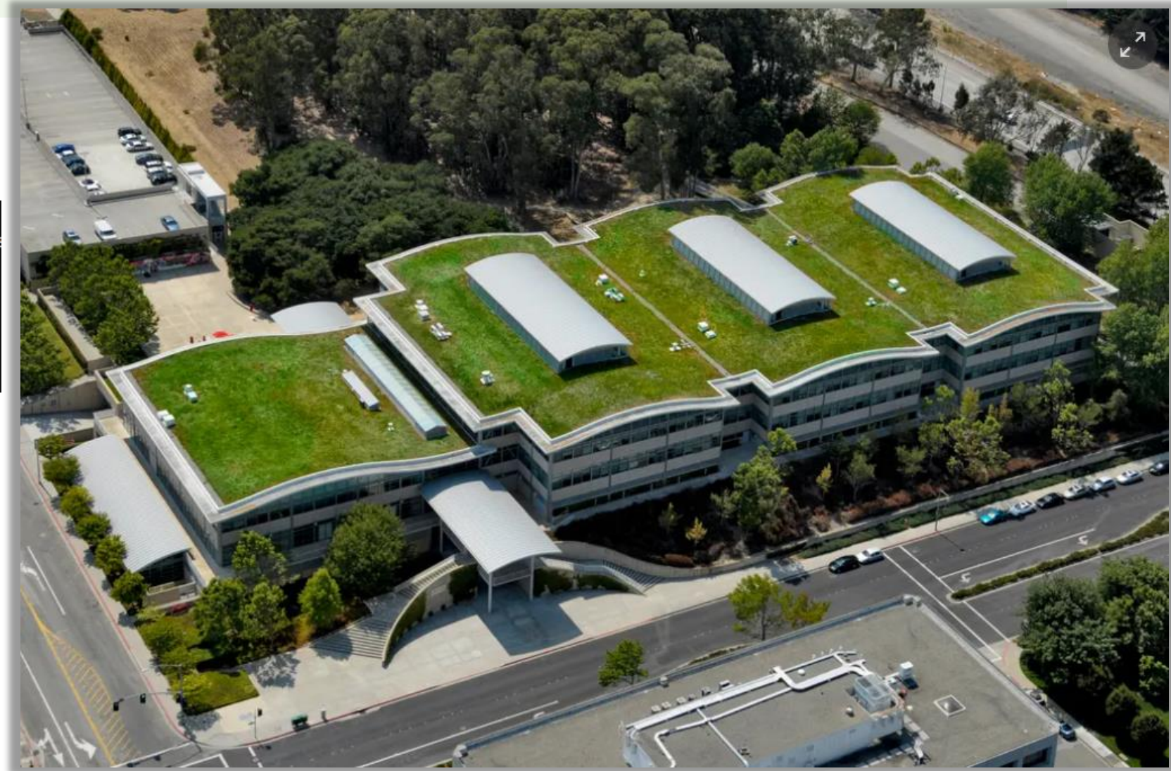
Gap's headquarters in San Bruno, California. Constructed in 1997, it is covered native indigenous grasses and wildflowers, cultivated from native grasslands in San Francisco. Photograph: Steve Proehl/Getty Images
